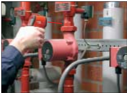
Checking supply and return flow to help determine efficiency of heating / cooling systems in seconds, not minutes.
